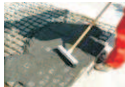
Sweep into the joints diagonally
