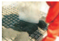
Spread material on the surface
