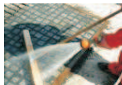
Clean the surface with soft jet of water
