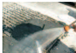
Increase density and prolong curing process by rinsing with soft jet of water
